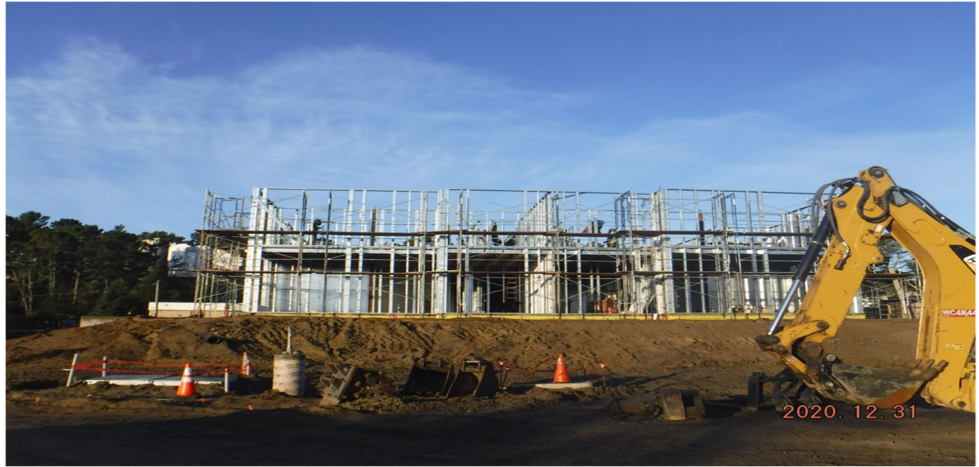
First and Second Floor Framing and Site Work
